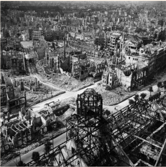
View from the Town Hall Tower over the destroyed city of Dresden
